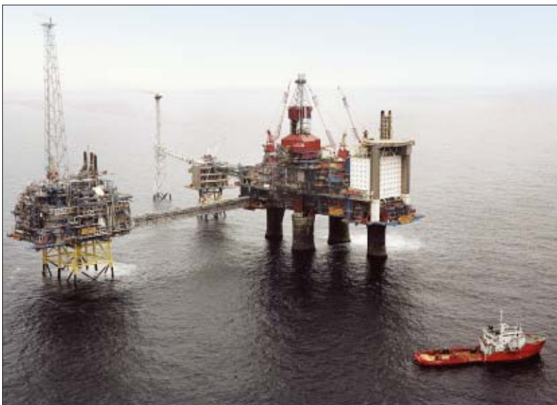
The Sleipner T gas treatment installation (left) linked by a bridge to the Sleipner A platform. (Photo: Øyvind Hagen.)
